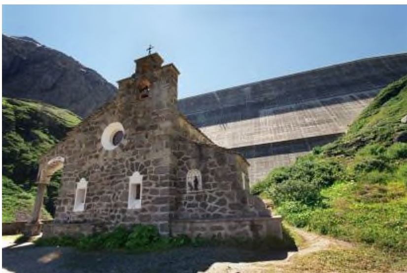
Staumauer Grande Dixence
