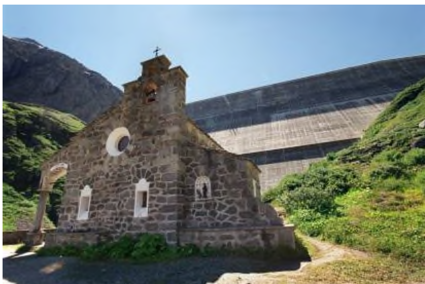
Staumauer Grande Dixence
