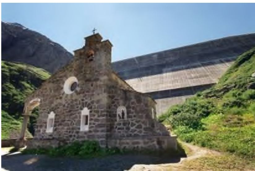
Staumauer Grande Dixence
