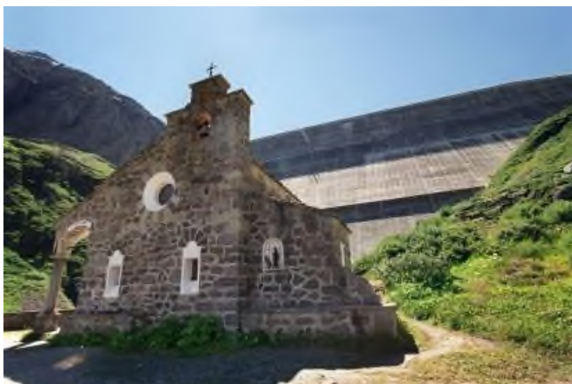
Staumauer Grande Dixence
